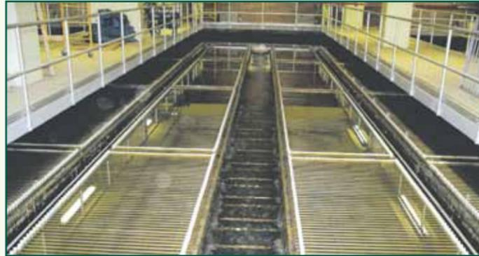
Sedimentation basin with inclined plates
