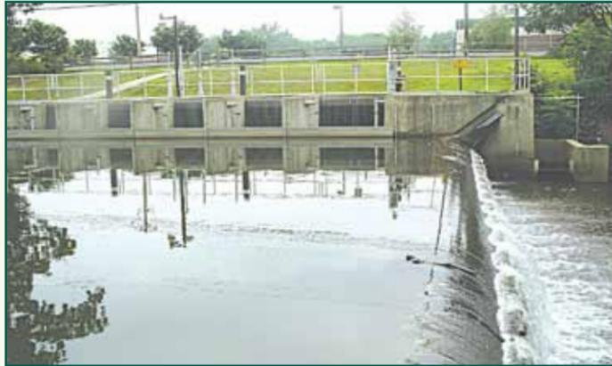
Raw water intake and inflatable dam
