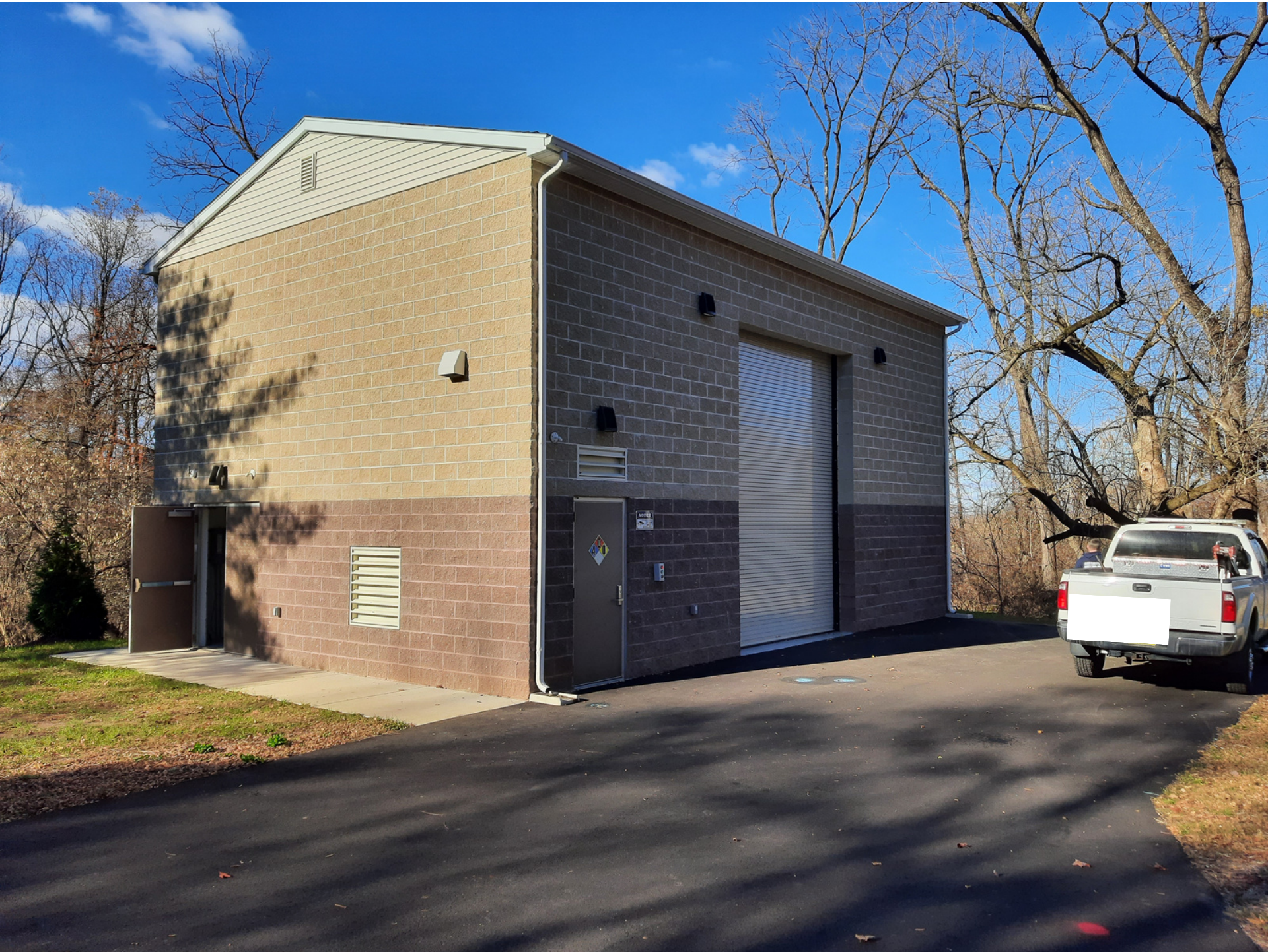
Building that houses filtration units for Well 11.
