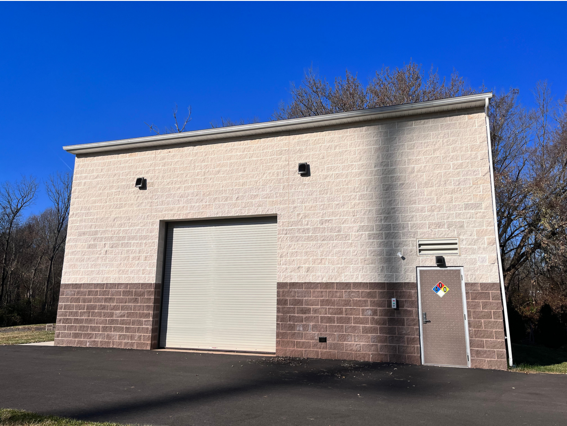
Building that houses filtration units for Well 3.
