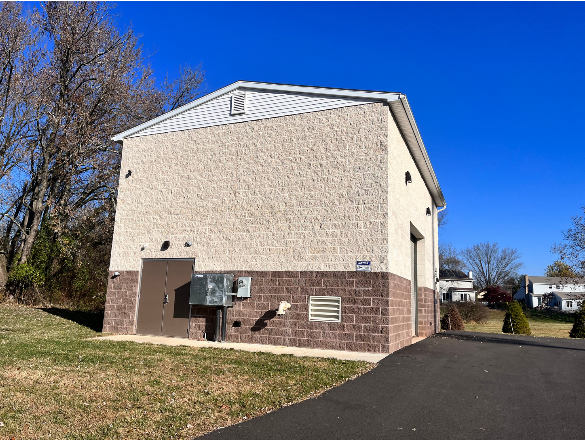
Building that houses filtration units for Well 3.
