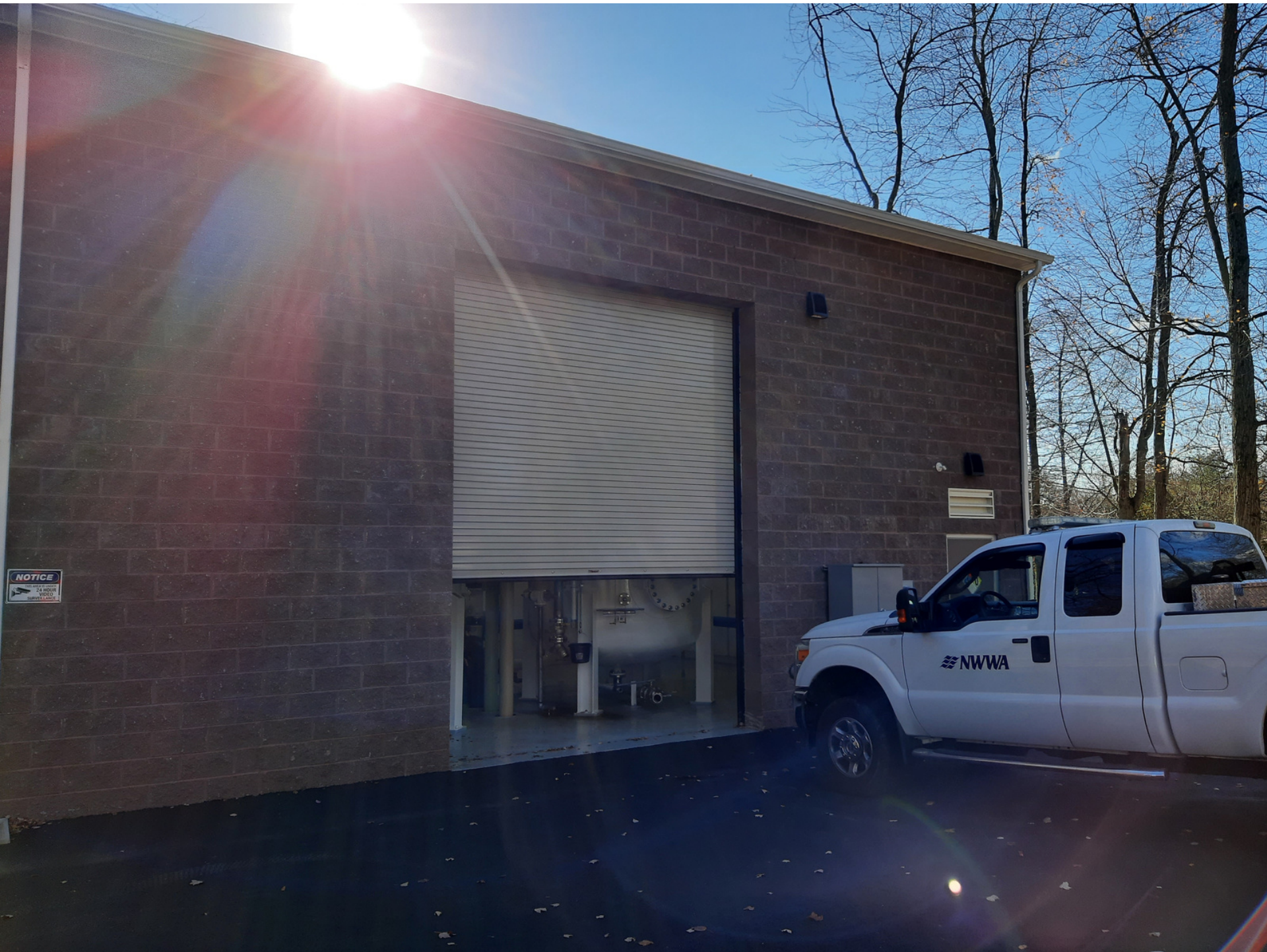
Building that houses filtration units for Well 5.
