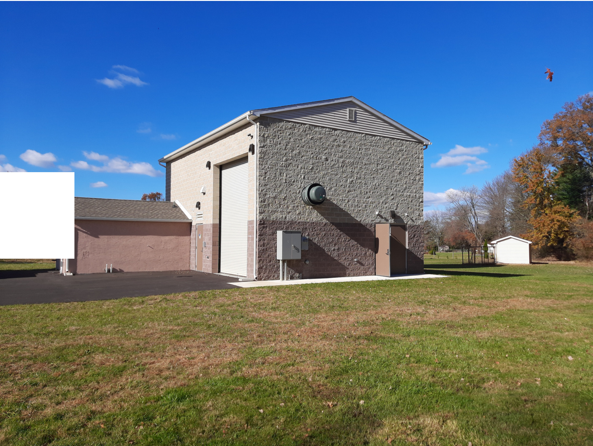
Building that houses filtration units for Well 8.
